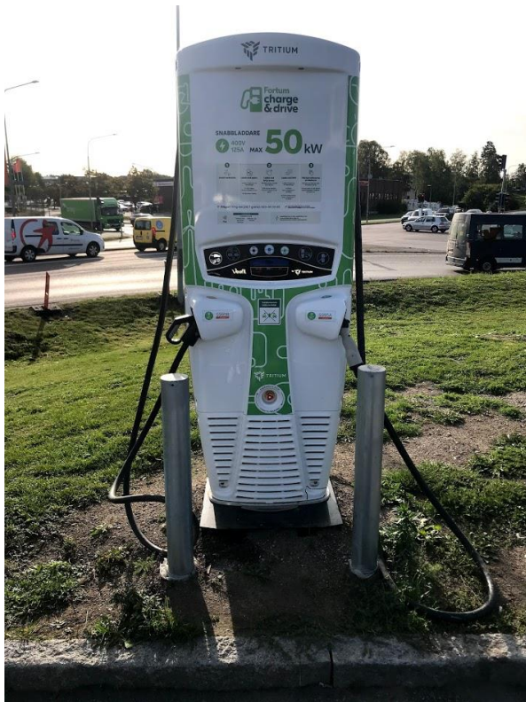
Tritium 50 kW station on Unimi-1baseQC including integrated protection bollards. This adaptor model is fastened via M12 anchors at the foundation sides. Protection bollards has been fastened by using drilled thru threaded rods + nuts
